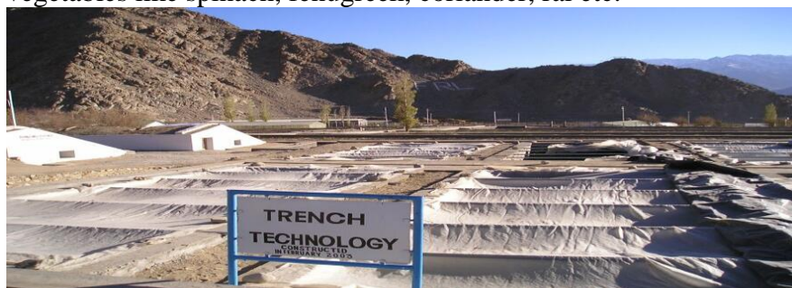
Fig 3: Trench Technology in Leh Ladakh
